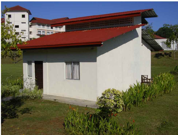
Figure 1. Structures made from OPS concrete. (a) Foot-bridge and (b) Low-cost house.
